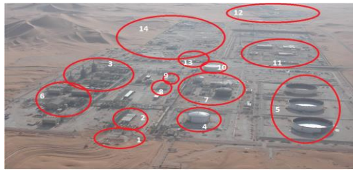
Figure 6: Succinct presentation of the production installations: General View of the CPF
